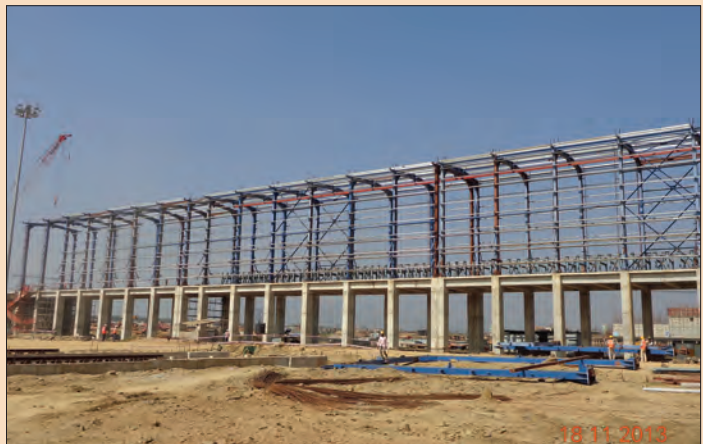
Steel fabrication works in progress at TATA Steel works, Kalinganagar
