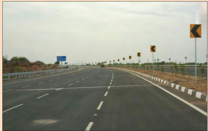
Hyderabad Outer Ring Road Project, Telangana
