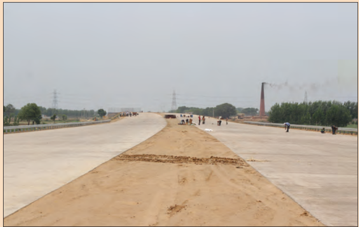
Road work in progress Six Lane Eastern Peripheral Expressway
