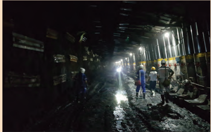
Under ground Mining work in progress at Jhanjra
