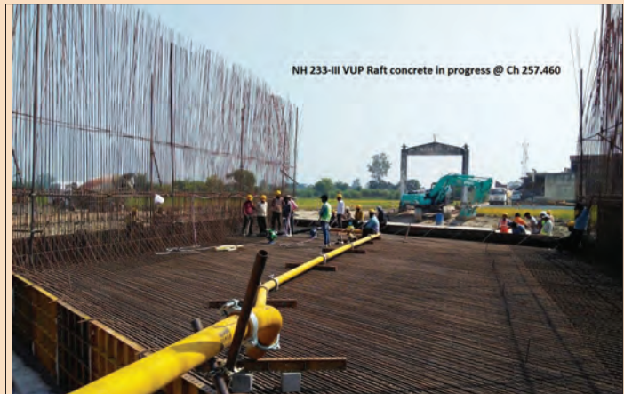
Raft concrete in progress at Varanasi
