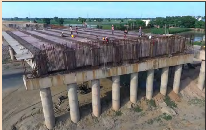
Road work in progress at Six Lane Eastern Peripheral Expressway
