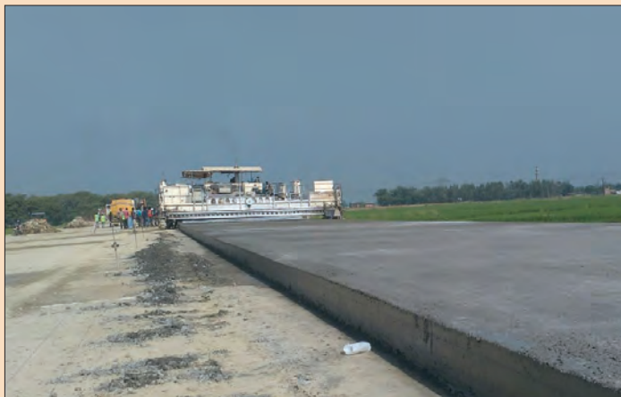
Cement Lining work in progress at Varanasi
